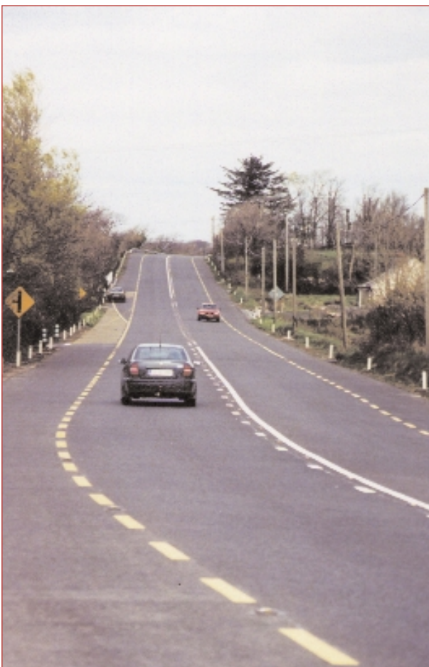
Newly aligned and surfaced section of the N15, north of Grange.
