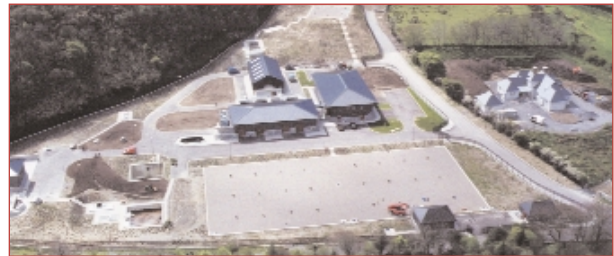
Treatment plant, Cairns hill.
